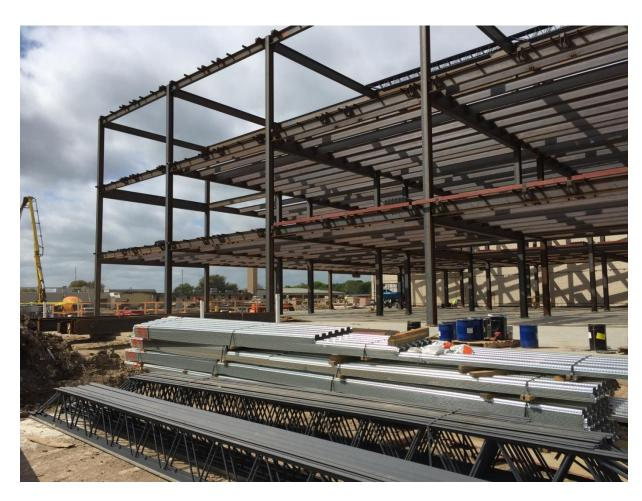
**ADMINISTRATION AND CLASSROOMS** – The steel structure erection is in progress on the 3 story classroom area. The administration offices are located on the first floor.
